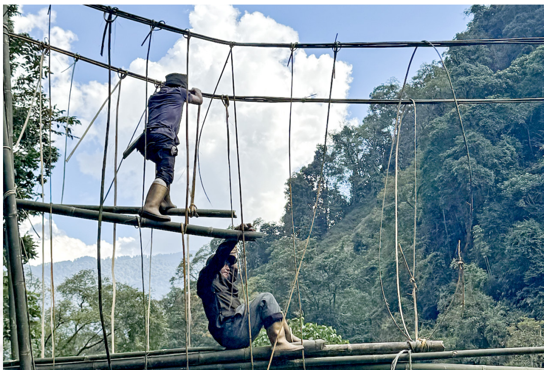
Tying the cane loops, with help of the soamvaa, 8 November 2025, JB
