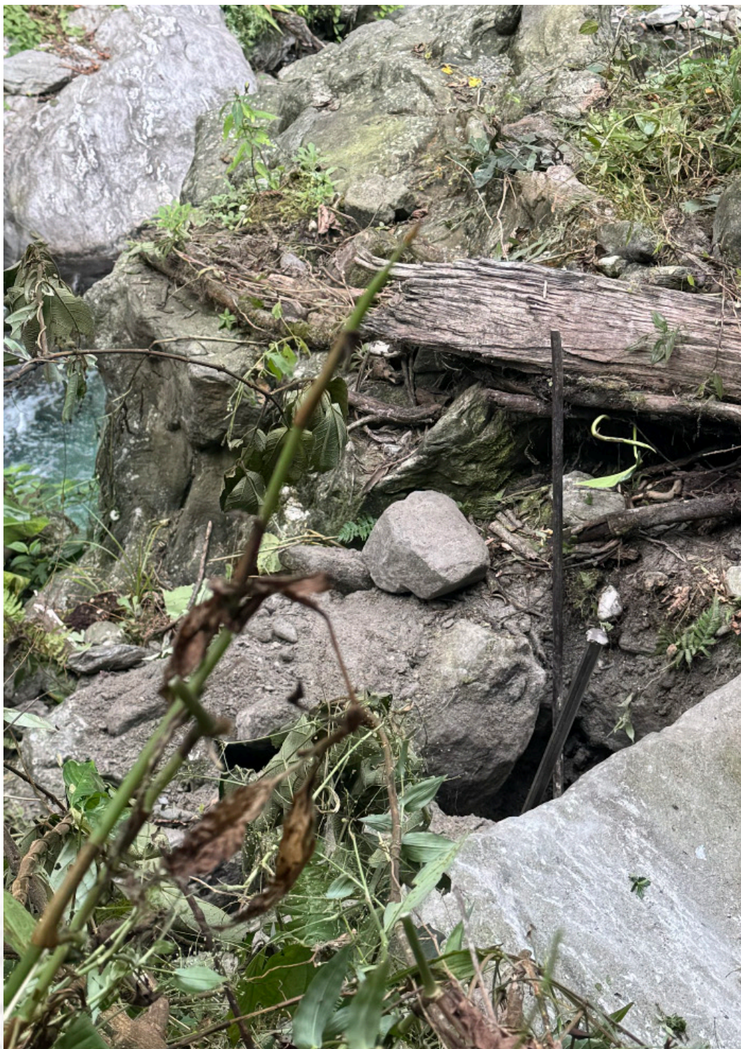
Digging the hole for the pillar, right riverbank, 6 November 2025, JB
