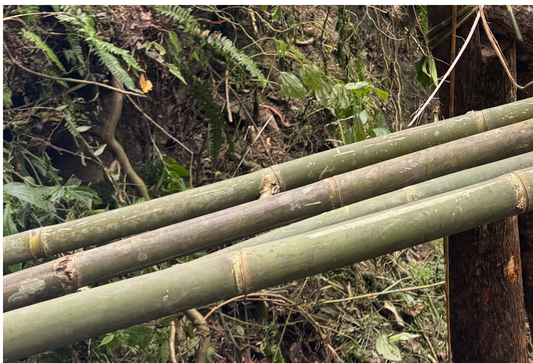
The bamboo used during bridge construction, 9 November 2025, JB
