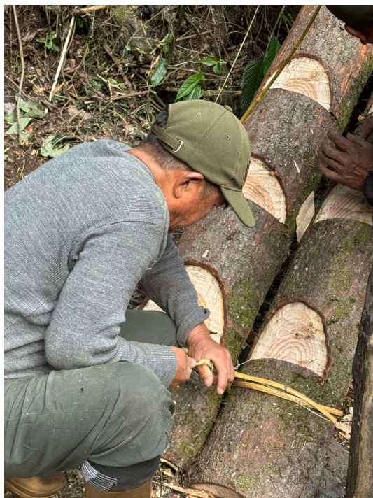
Tying the wooden stairs with cane, 10 November 2025, JB
