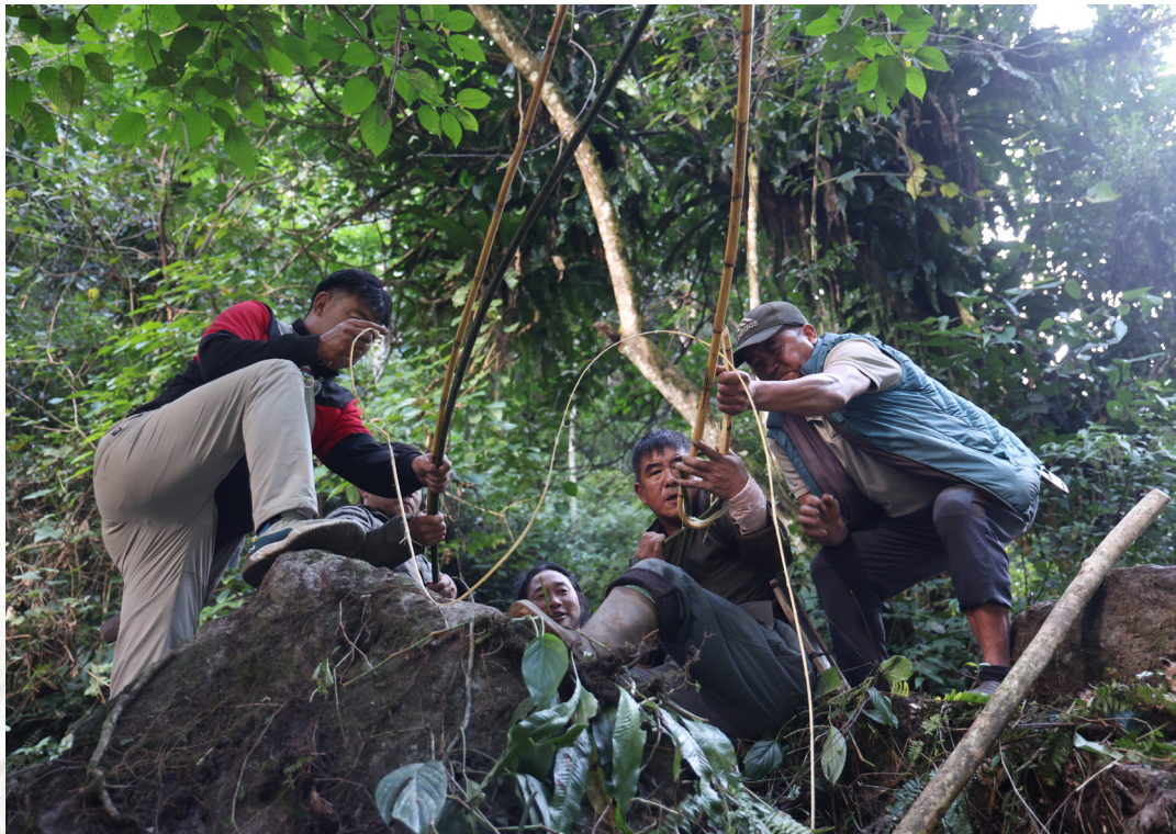
Pulling the suspension cane vines (soamglyaang) over the river, 7 November 2025, PP
