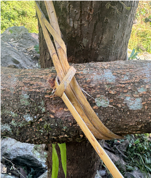
Knots. To make the knot more durable, the cane is twisted. 8 November 2025, JB
