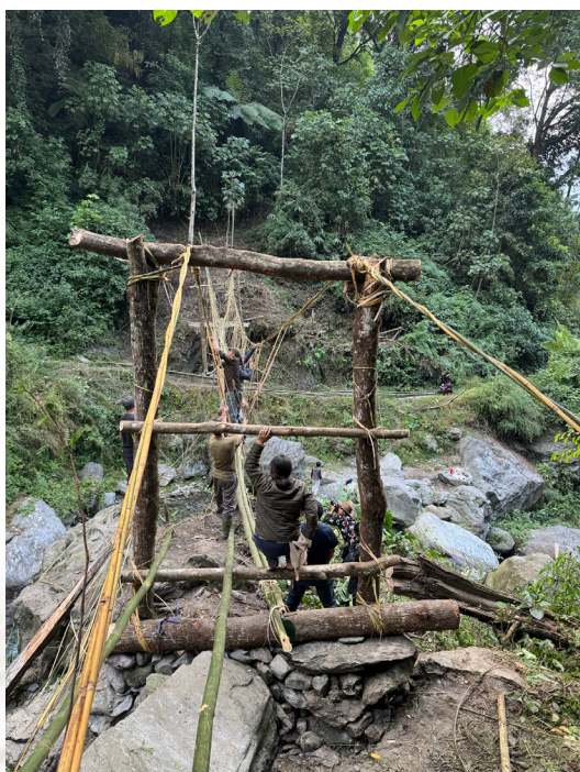
Tying the bamboo to the pillar structure, securing the bridge on the opposite side, 9 November 2025, JB
