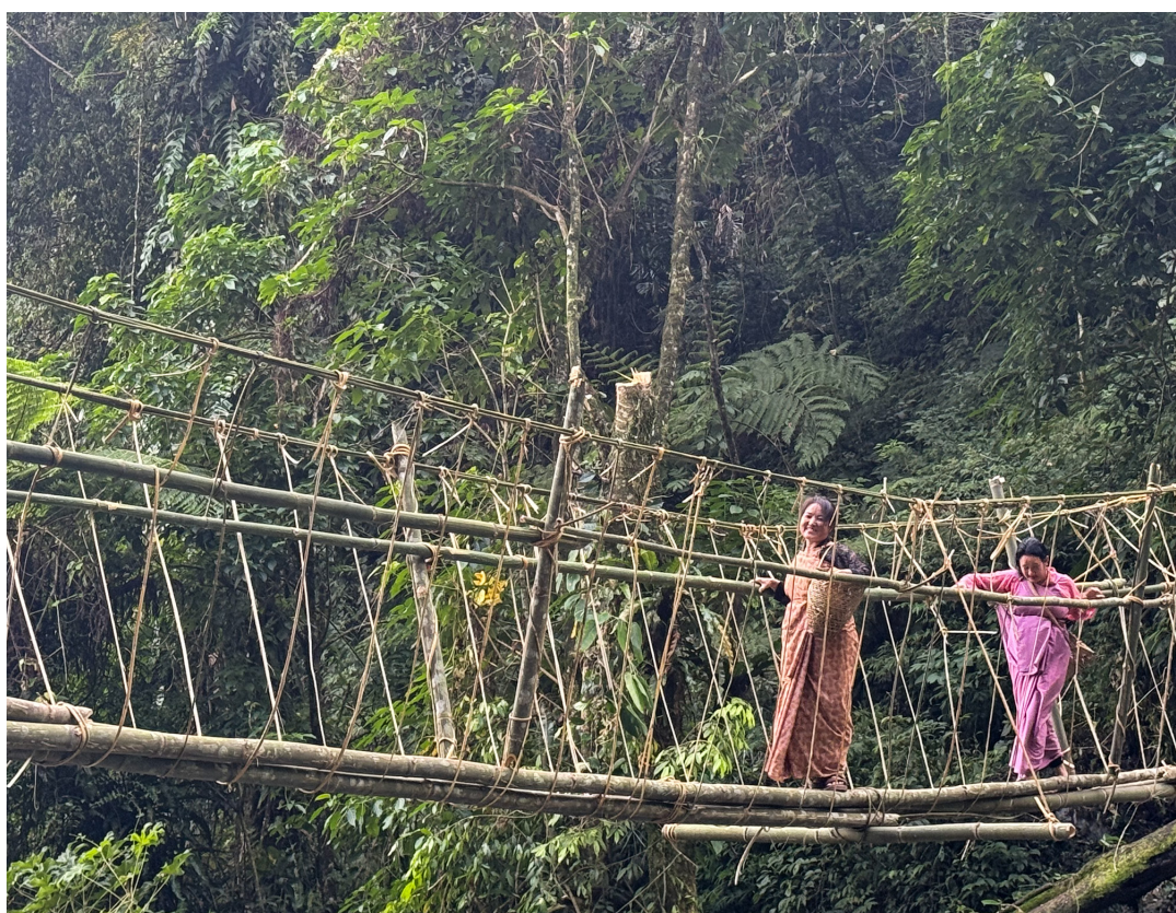
Safe crossing of the bridge, 11 November 2025, JB
