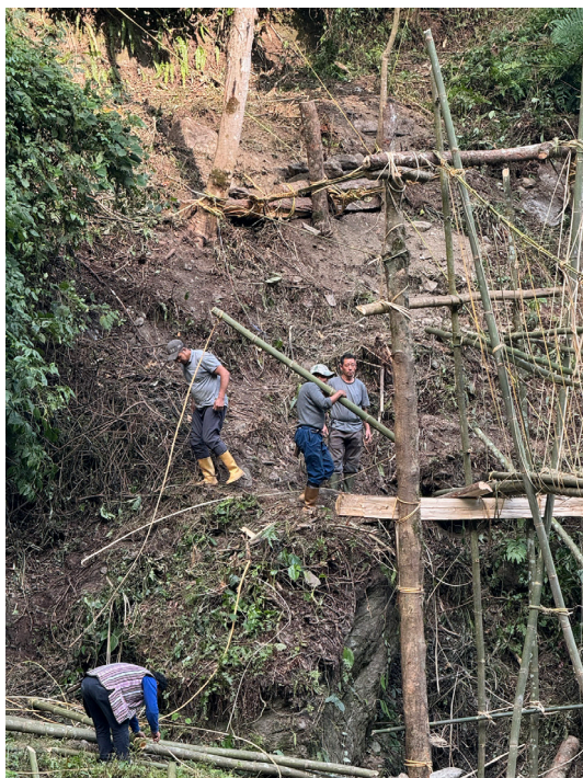
Special structure, soamlook tukvyaa, to prevent the bridge from caving in, 9 November 2025, JB
