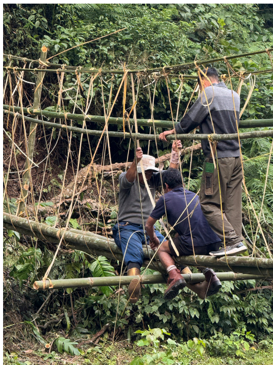
Special structure, soamlook tukvyaa, to prevent the bridge from caving in, 9 November 2025, JB
