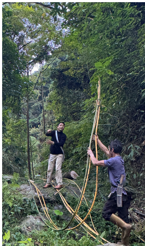
Pulling from the other side, attaching the second suspension cane vine bundle, 7 November 2025, JB
