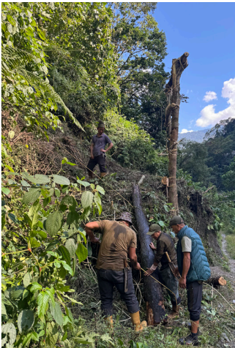
Making the beam structure to attach the suspension cane vines, 7 November 2025, JB
