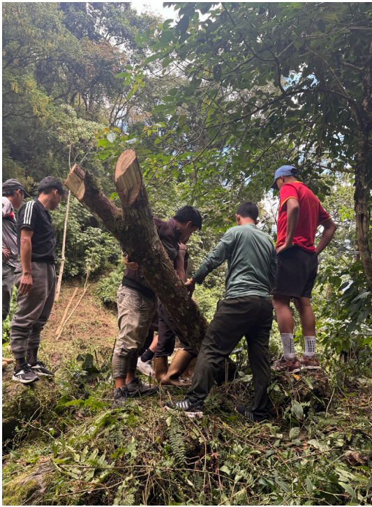
Lifting the tree trunk into the hole, and adjusting the pillar, 6 November 2025, JB
