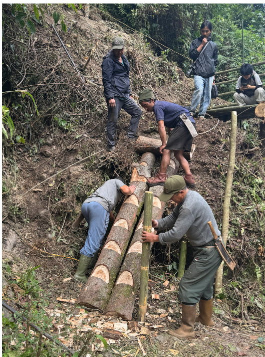
Tying the wooden stairs with cane, 10 November 2025, JB
