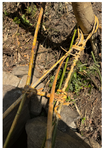
Additional cane support for the soamglyaang, 10 November 2025, JB
