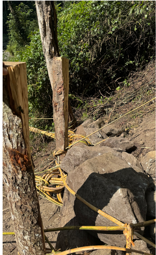
Strengthening the supporting structure, 8 November 2025, JB; stones over the tree trunk and increased cane support, 9 November 2025, JB
