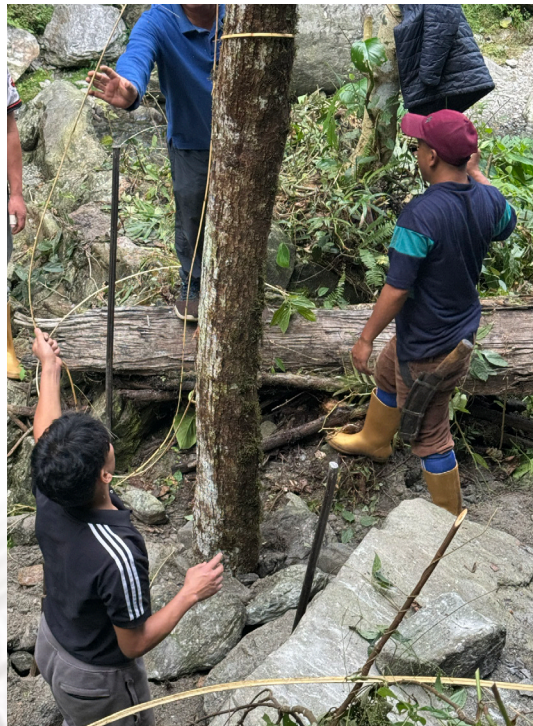
Stabilising the pillar with stones, 6 November 2025, JB
