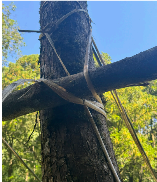
Knots. To make the knot more durable, the cane is twisted. 8 November 2025, JB
