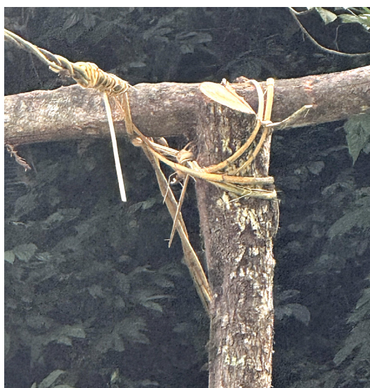
Tying the suspension cane vines to the pillar structure, 8 November 2025, JB
