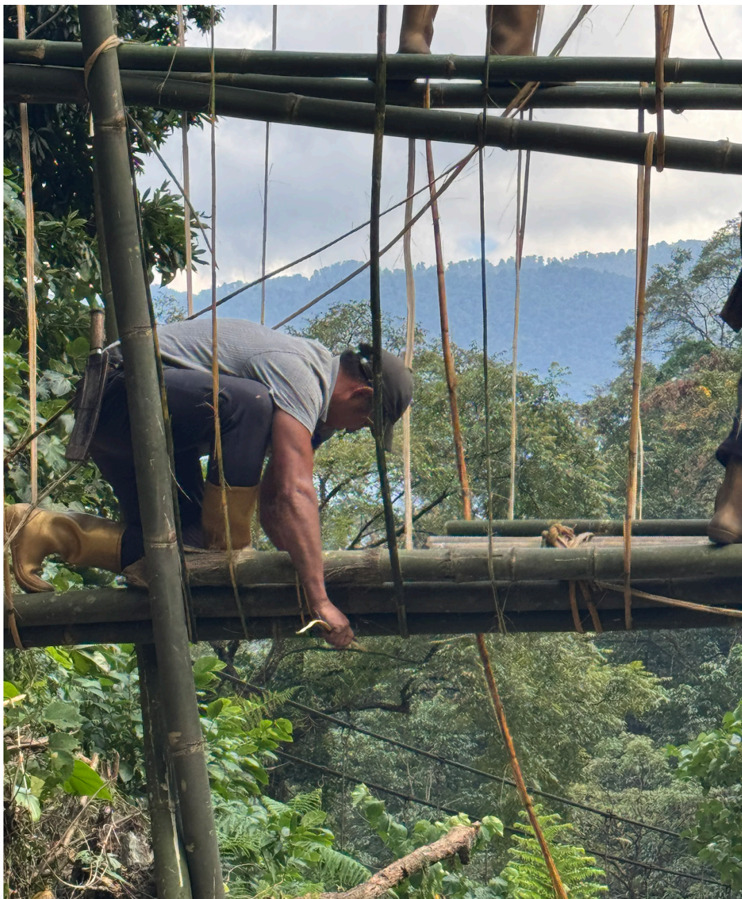
Tying the soamvaa to the bamboo for stability, 8 November 2025, JB
