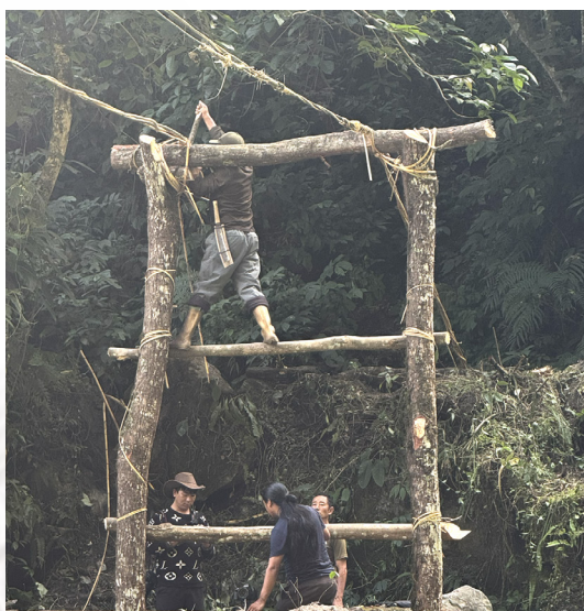
Tying the suspension cane vines to the pillar structure, 8 November 2025, JB
