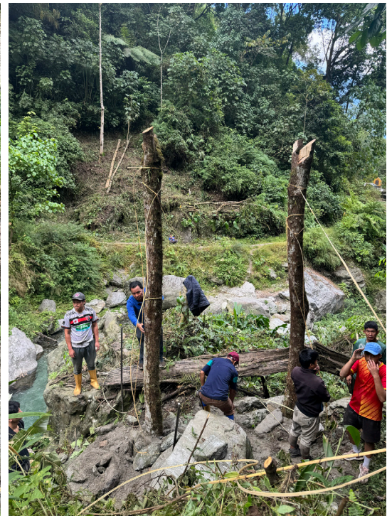
Stabilising the pillar with stones, 6 November 2025, JB
