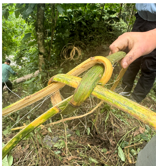
Tying the crossbeam; close-up of a knot in cane, 6 November 2025, JB
