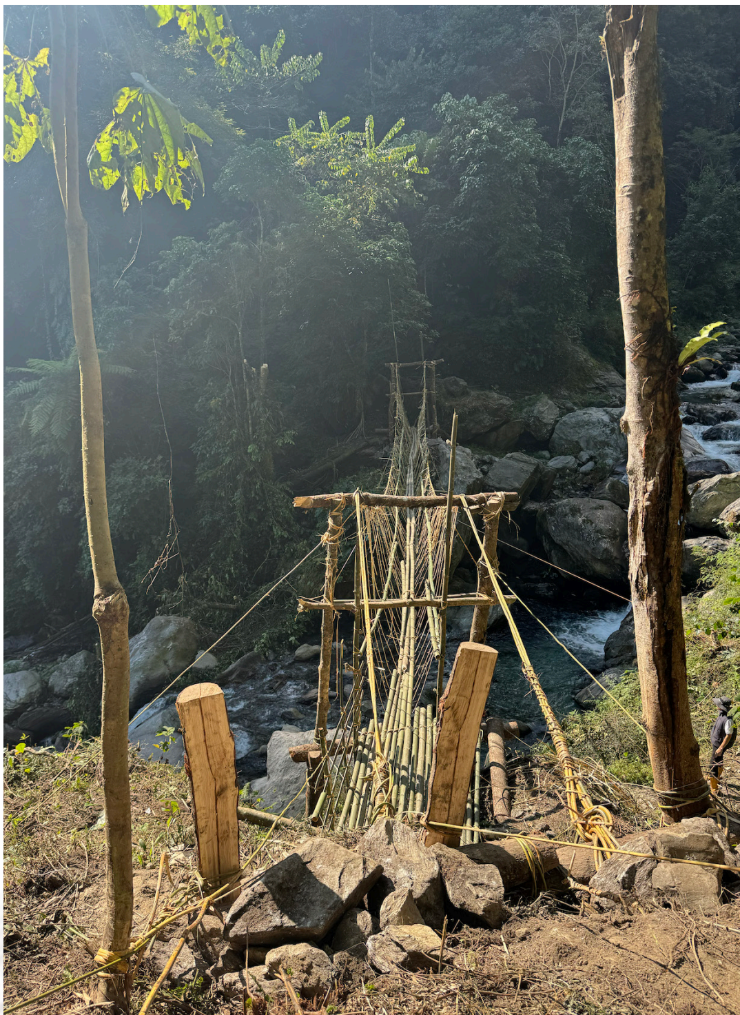
View from above with the crossbeams, pillars, and stones holding the suspension cane vines in the foreground, 9 November 2025, JB
