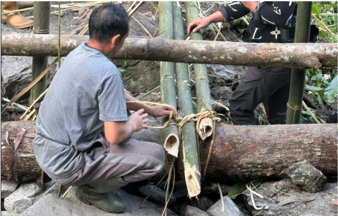
Tying the three bamboos for walking on to the log crossbeam, 9 November 2025, JB
