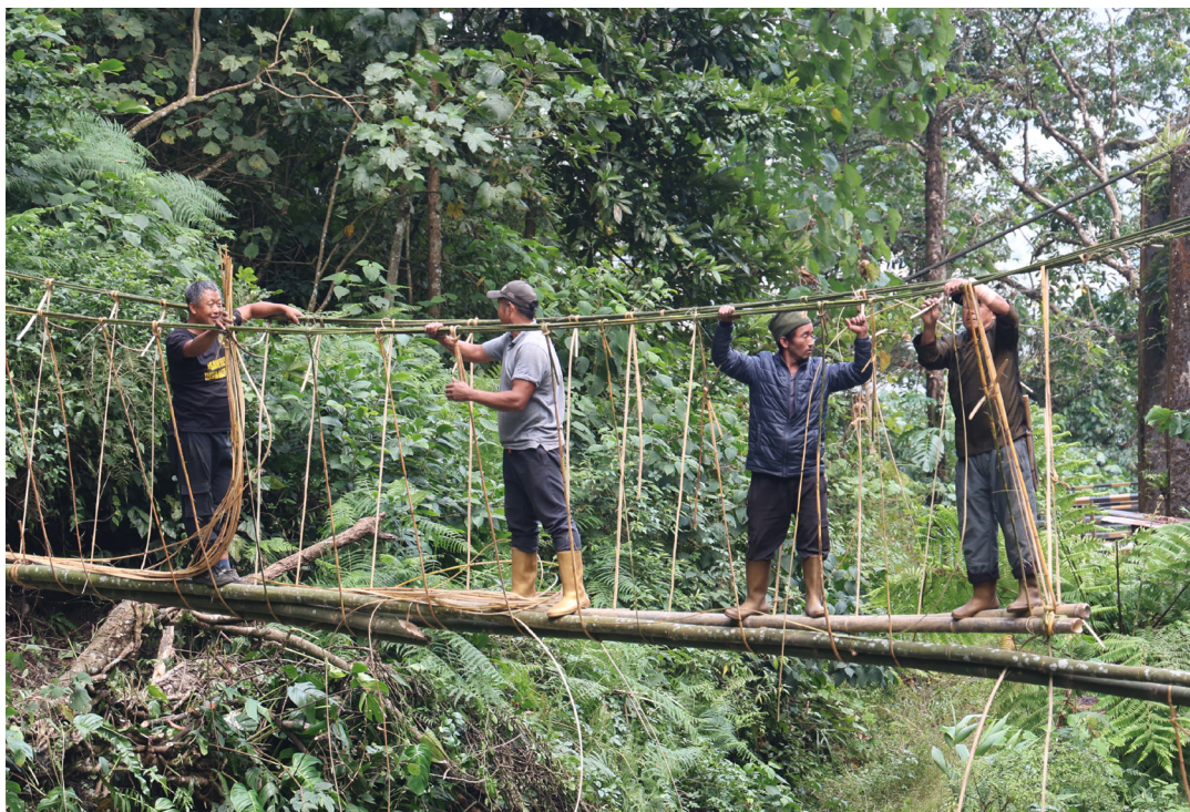
The soamnoakboo (master builder) ahead, the chhaakokorboo (main helper with the loops) and the other helpers, maximum 4 people are on the bridge while building, 8 November, PP
