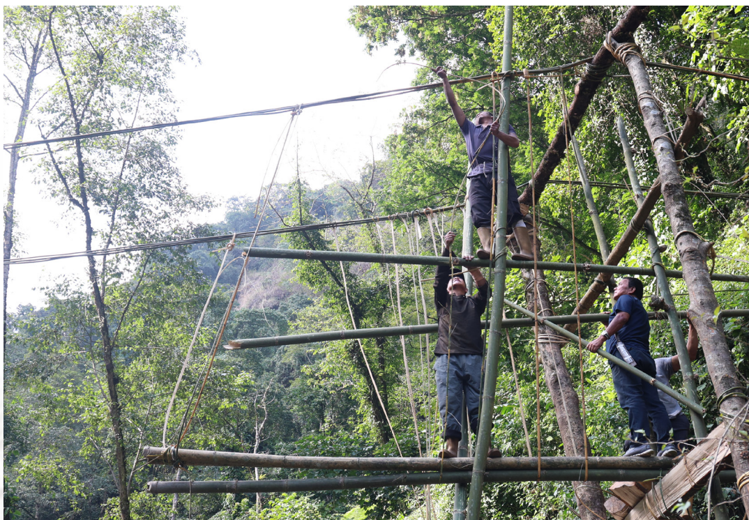
Passing the cane loops up to tie the knot, 8 November 2025, PP
