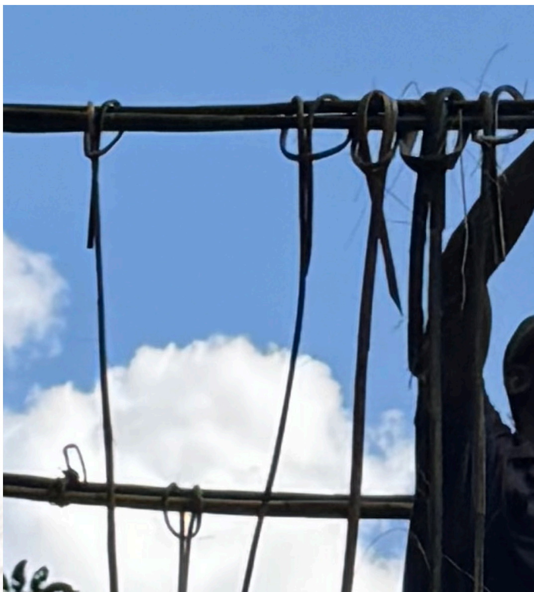
Aatyaap, specialised knots for bridge building, 8 November 2025, JB
