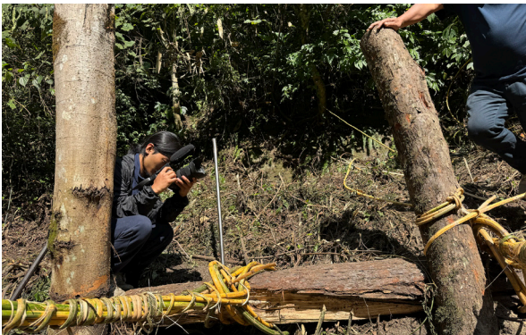
Again, additional cane is twisted around to make sure the knots do not open, 8 November 2025, JB
