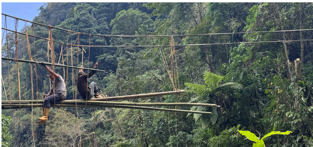
The loops attached to the soamvaa have just been tightened the second time, 8 November 2025, JB
