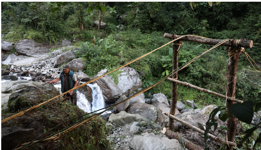
The suspension cables are laid across the soamglyaang tingbo, 8 November 2025, JB
