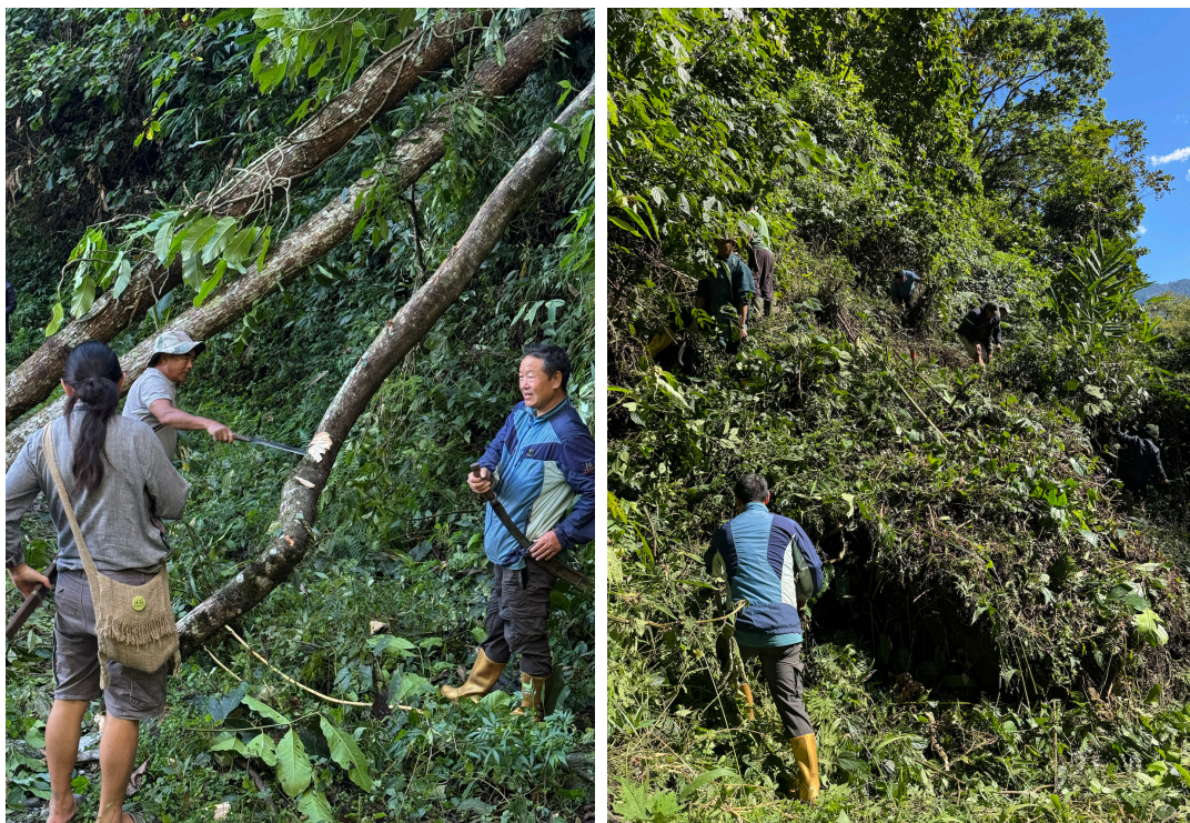
Clearing the area, cutting the trees, 4 November 2025, JB
