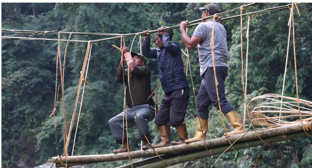
Tightening the loops, 8 November 2025, PP
