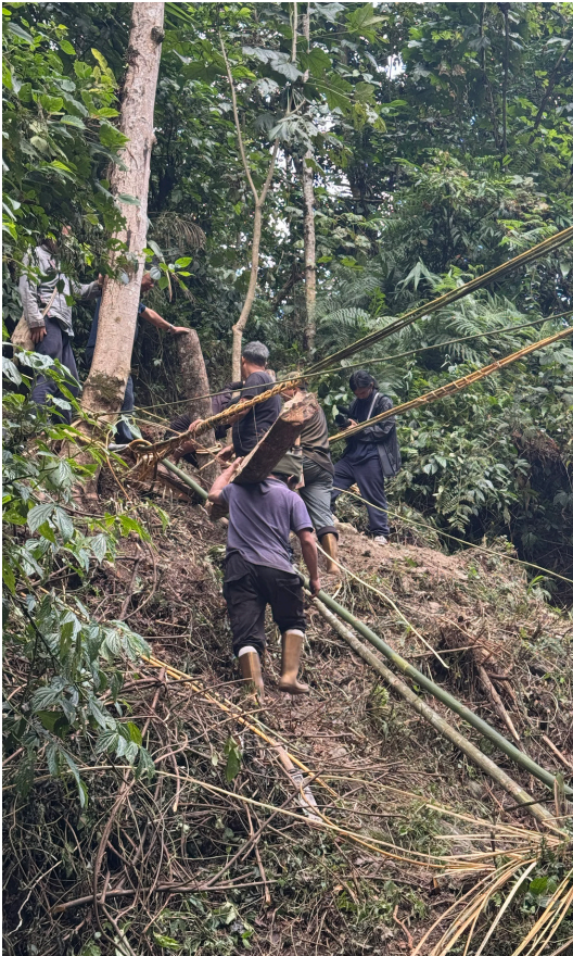
Strengthening the supporting structure, 8 November 2025, JB; stones over the tree trunk and increased cane support, 9 November 2025, JB
