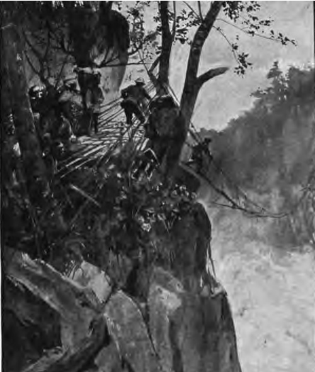
Bridge at Samdong, Waddell 1900
