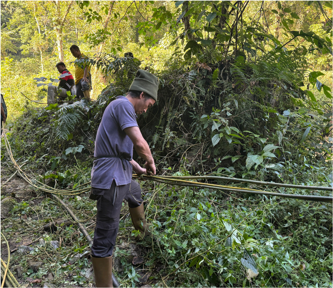
Bundling three canes to make the suspension cane vine, 7 November 2025, JB
