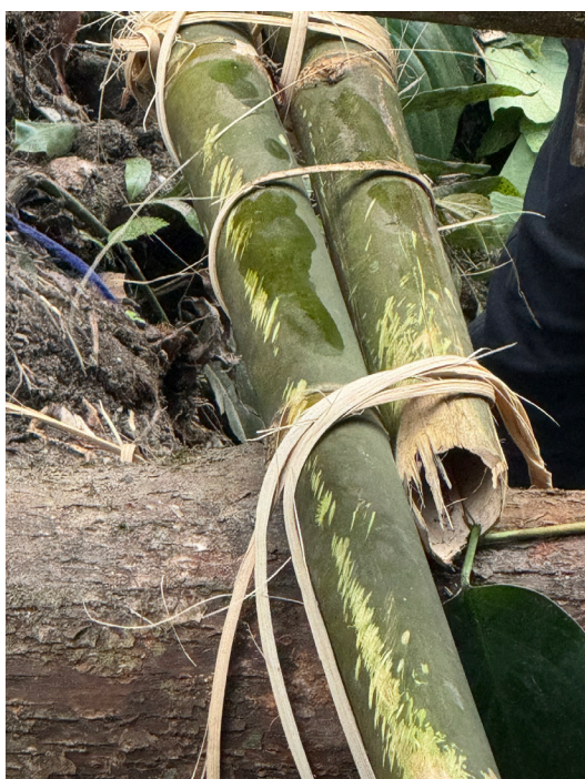
Tying the bamboo to the pillar structure, securing the bridge on the opposite side, 9 November 2025, JB
