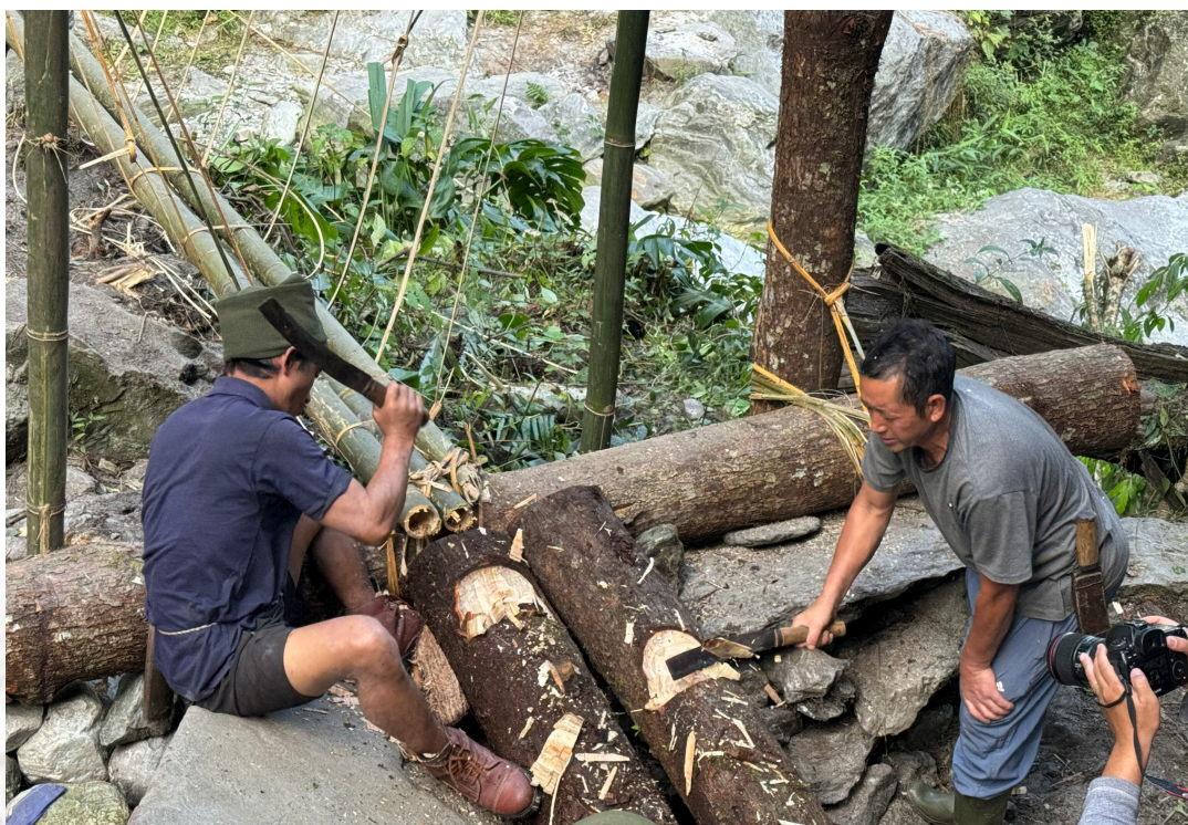
Making a stairs to reach the bridge, 10 November 2025, JB
