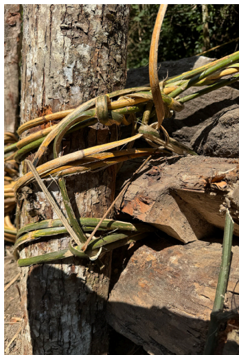
Additional cane support for the soamglyaang, 10 November 2025, JB
