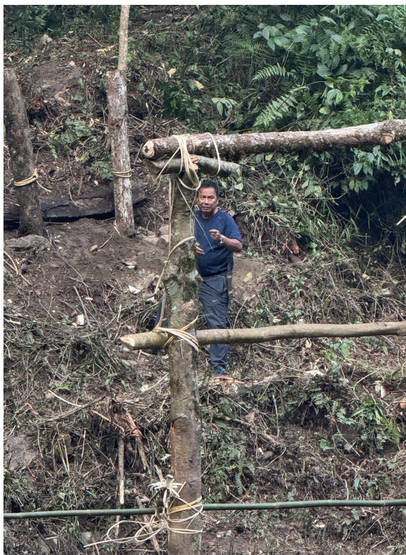
Pulling from the other side, attaching the second suspension cane vine bundle, 7 November 2025, JB
